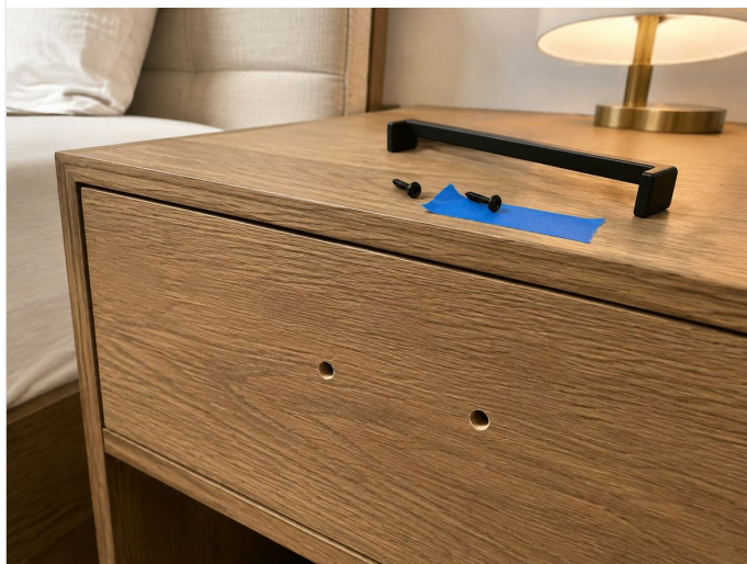
Room 204 nightstand — missing pull hardware
